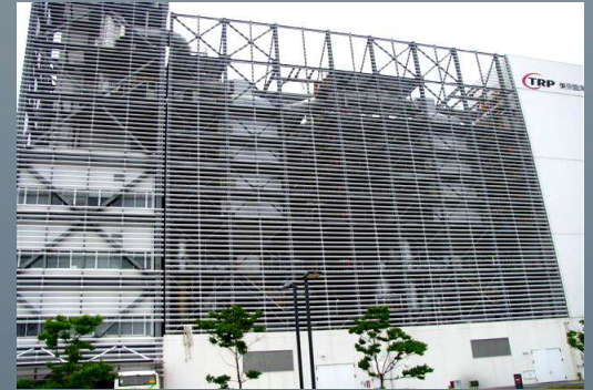
Gasification Plant Tokyo, Japan
