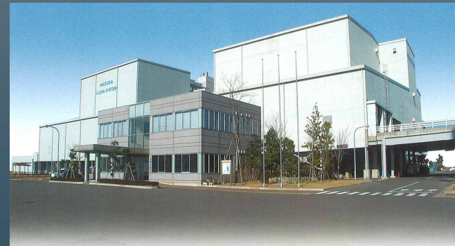
Kazua Clean System Co., Ltd. Gasification Plant - Japan
