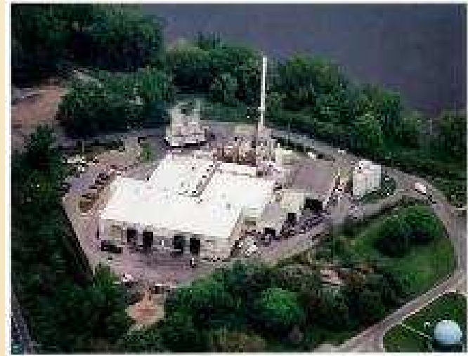
408 Ton per Day WTE Facility in Agawam, MA.
