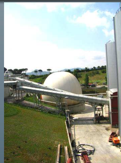
Anaerobic Digestion of MSW Barcelona, Spain
