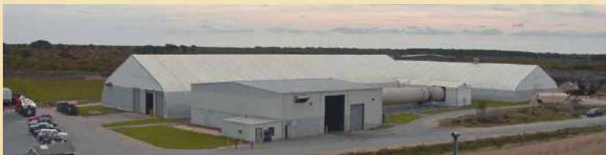
Mixed Waste Composting Facility in Nantucket, MA
