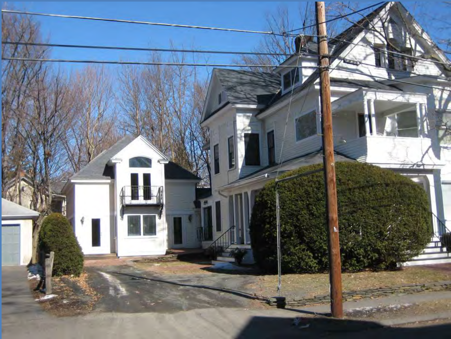
CARRIAGE HOUSE CONVERSION, BUTLER PLACE
