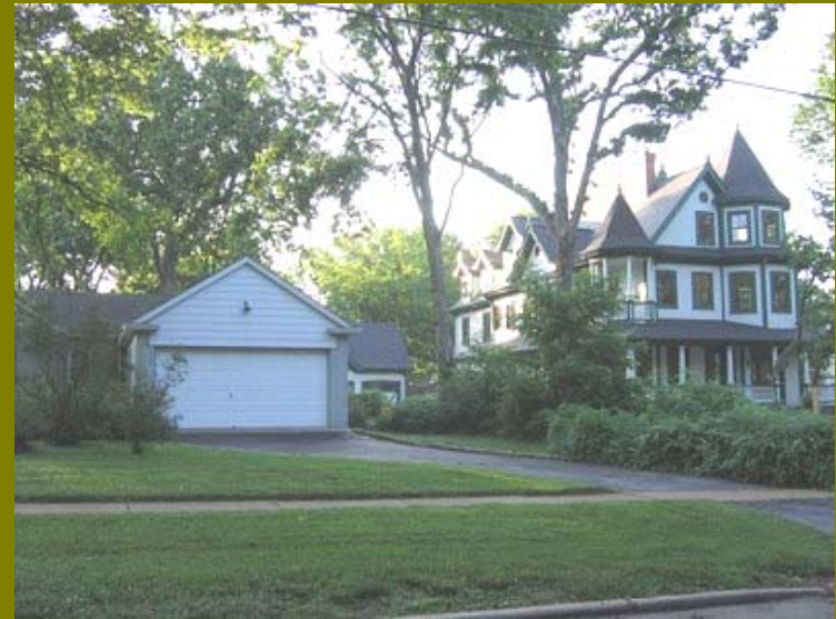
This garage-dominant, neo-eclectic design does not relate to the adjacent historic buildings.
