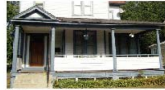
Typical wrap around porch with hip roof and gable accent over the stairway
