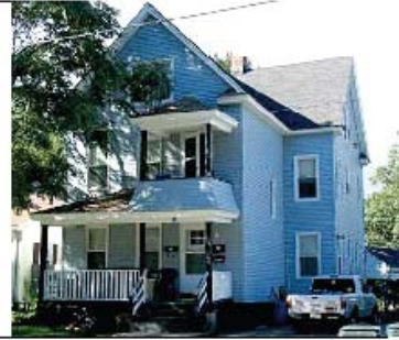
The double-decker porch is a common feature on Springfield Gable Vernacular homes and duplexes.
