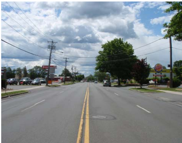
King Street View South – Before
